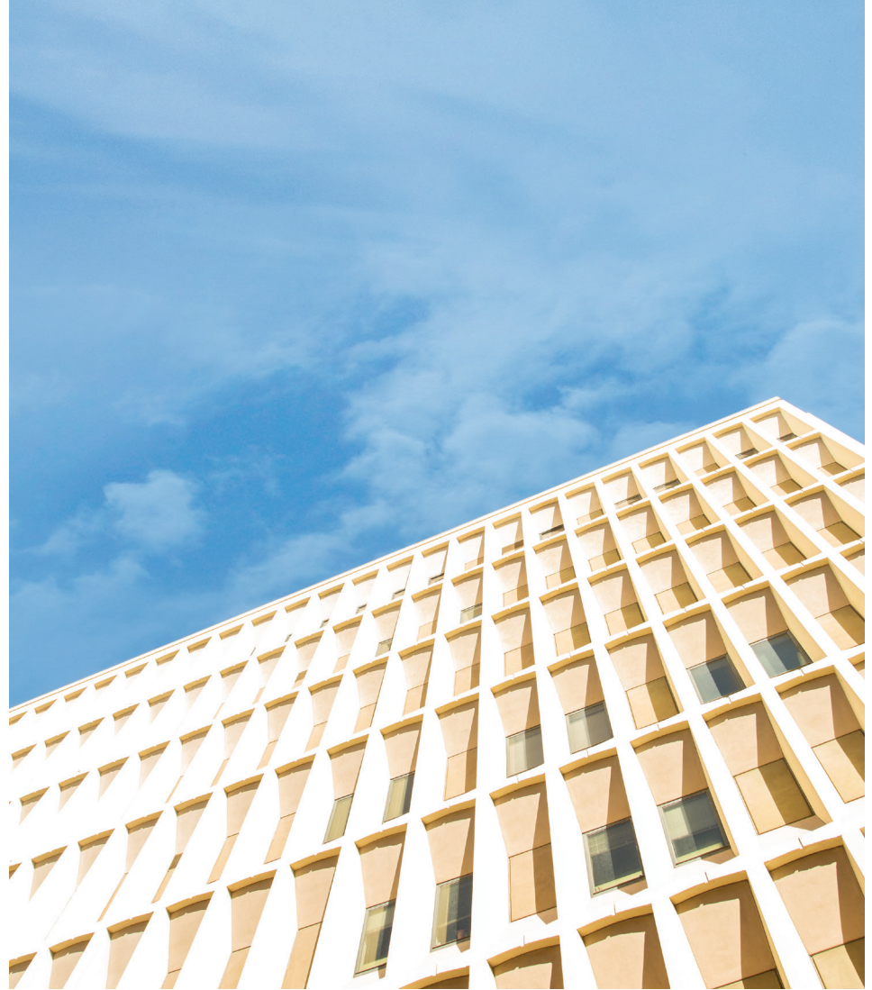
Franz Hall is one of three UCLA Psychology buildings that will be modernized and upgraded as part of a new $150 million capital project.
