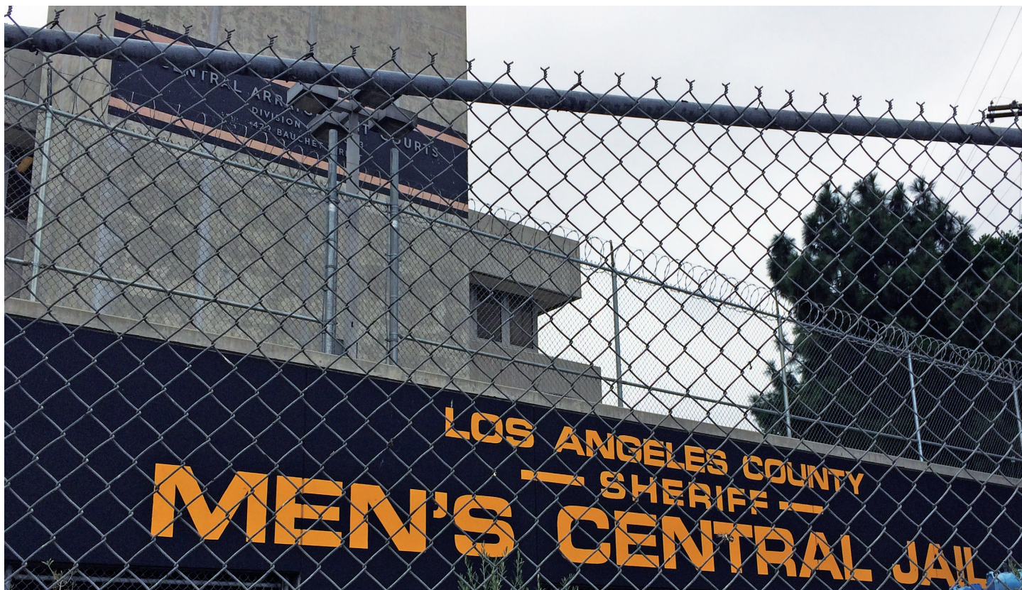
Los Angeles County Men's Central Jail in downtown. Los Angeles operates the largest jail system in the United States.
