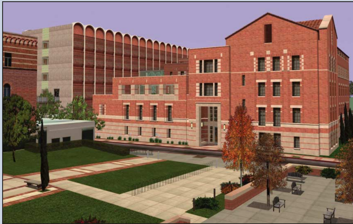
The College's new Physics and Astronomy Building, attached to Knudsen Hall due south of Powell Library, will house state-of-the-science laboratories and classrooms.
